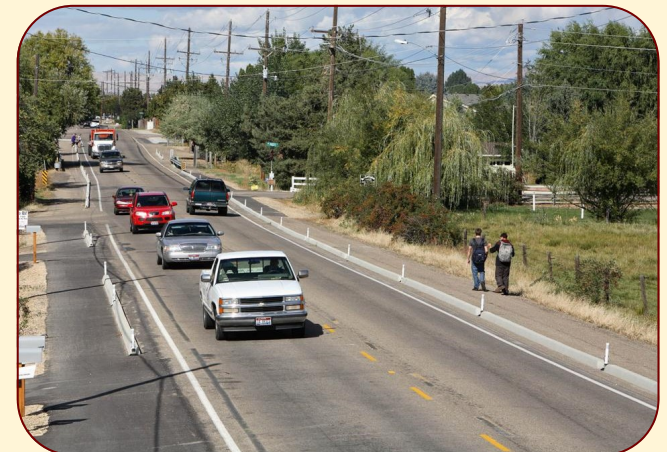
F: Shoulder/extruded curb pathway in Ada County, ID (constructed with federal Safe Routes to School funds)
